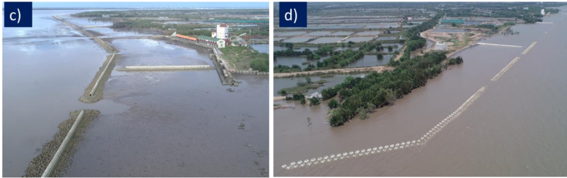
Figure 6. The prefabricated components of TC1 (a) and TC2 (b) in the factory and installation on the construction field in Con Cong (c, d), Tien Giang 2020
