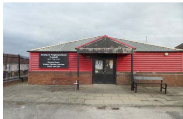
Figure 1. Front view of the building
