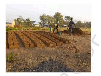
Fig. 2. Reddish Clayish soil used for plaster and blocks preparation in Wa, 2022 (photograph by the authors).
