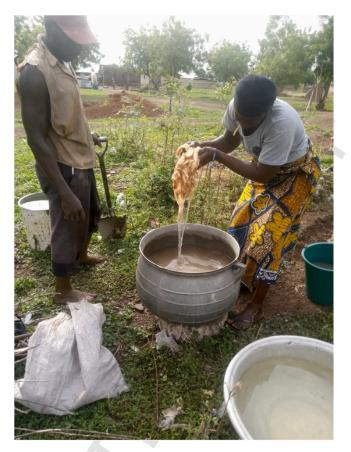
Fig. 7. Mixing shredded beini roots in water to prepare the biostabiliser solution (photograph by the authors).
