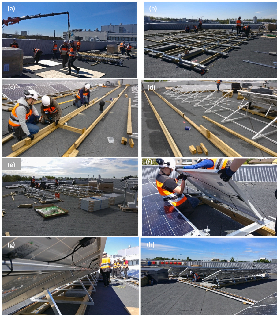
Fig. 8. Critical process stages in PV system deployment including construction and installation.
