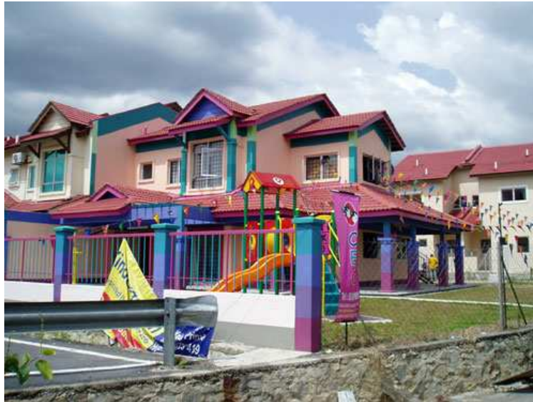
Figure 3. Double storey link house refurbished as a kindergarten
