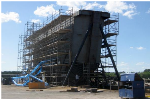
Figure 4.8: Dry dock gate construction
