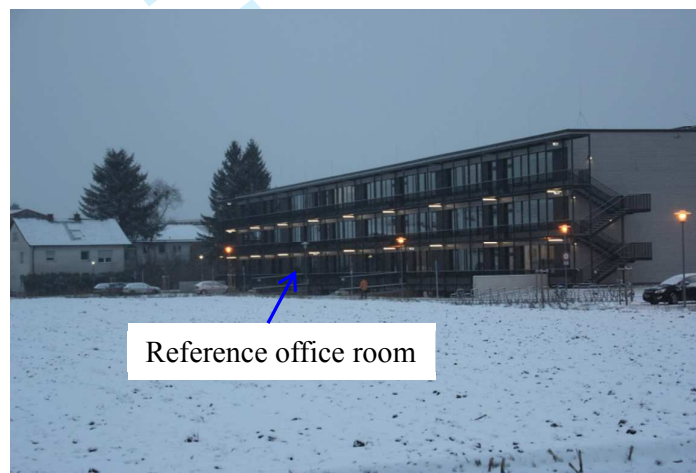
(b) North façade of new low-energy school building and the reference office room
