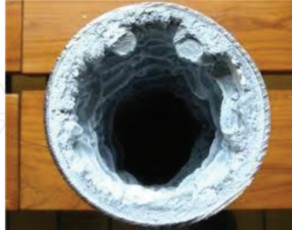
Figure 4. Heavy build-up of deposition on heat exchanger piping [24][23].
