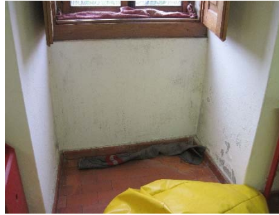
Figure 14 - Detail view from the interior showing the wood window and the thickness of exterior walls.
