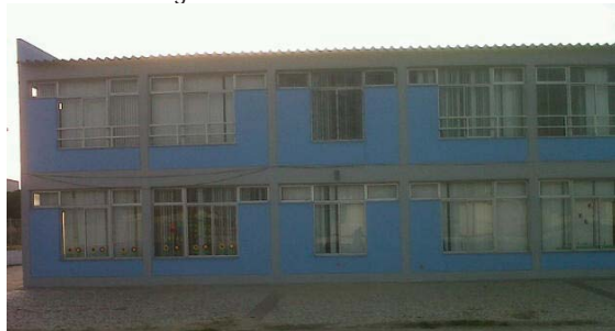
Fig.7: East view of one of the buildings.
