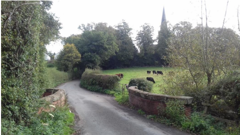
The bridge on Church Lane, with St John the Evangelist Church in background
