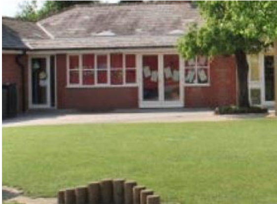
Image 6.1 - School A, showing classrooms surrounding one of the play areas (School A School website, n.d.)
