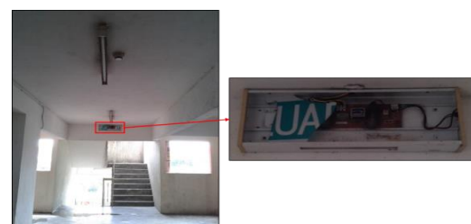
Figure 13: Vandalized emergency exit sign
