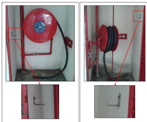
Figure 11: Missing portable fire extinguishers
