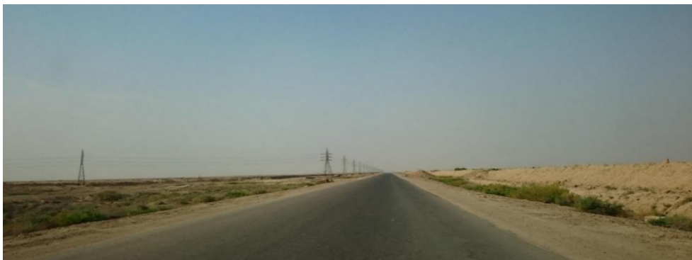
Figure 7.17: The area surrounding the pipelines.
