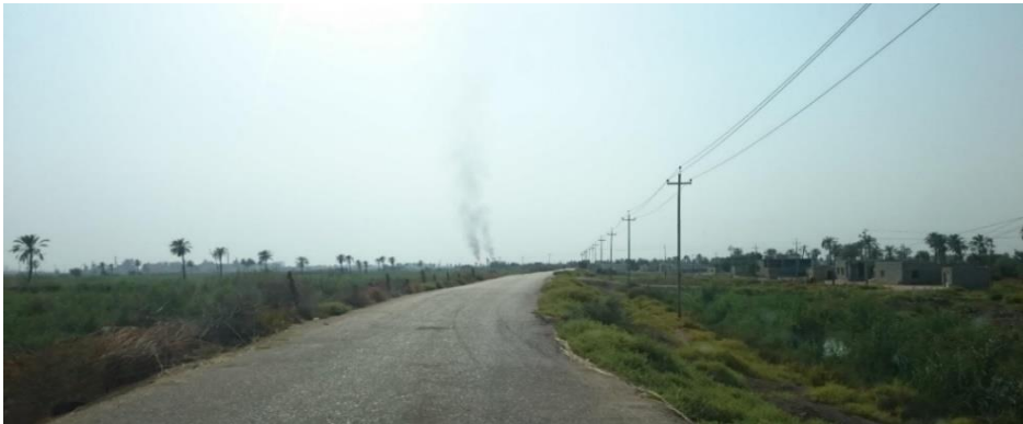
Figure 7.13: Green area and road crossing of section 1 of route 1 of the pipeline
