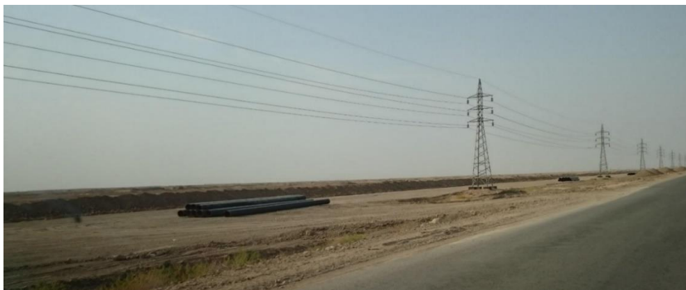
Figure 7.19: The area surrounding the pipelines.
