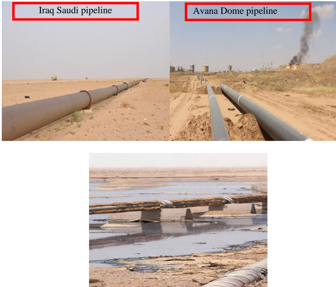
Figure 1.4 Examples of above ground pipelines in Iraq. Photos of Iraq’s pipelines (Walt, 2009; Adel, 2013).
