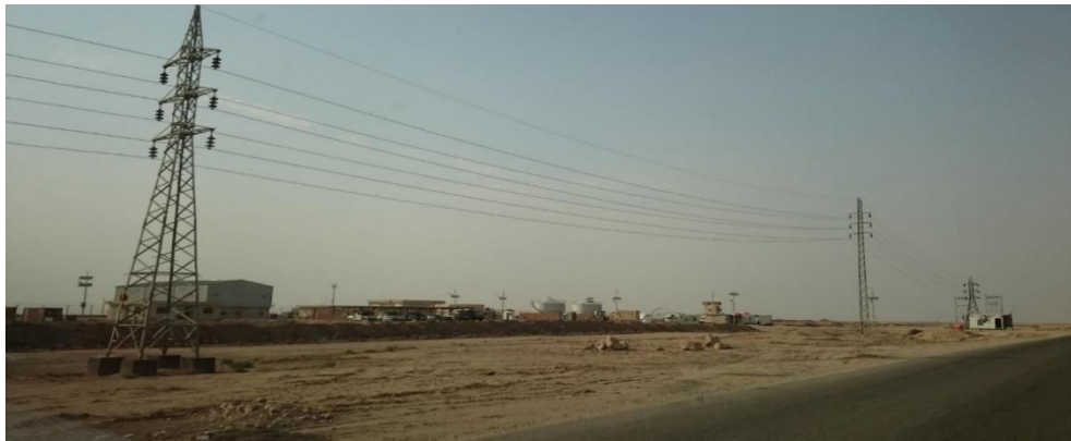
Figure 7.18: The area surrounding the pipelines.
