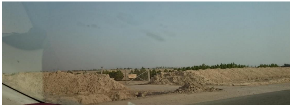
Figure 7.16: The area surrounding the pipelines.
