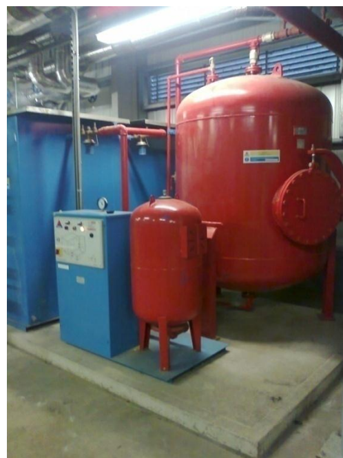
Fig 1. MTHW primary circulation pumps and pressurisation units – The Royal Derby Hospital
