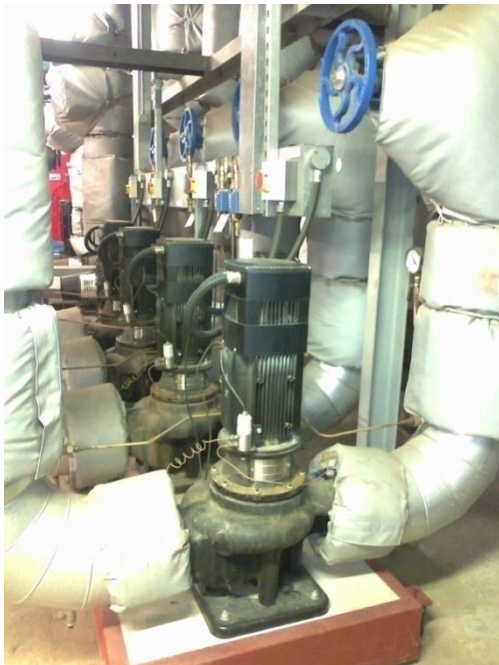
Fig 1. MTHW primary circulation pumps and pressurisation units – The Royal Derby Hospital
