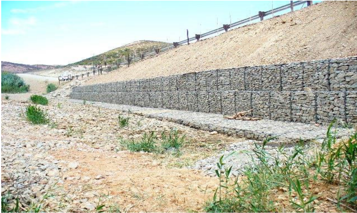
Figure 1.2: Gabions used for scour protection along embankment
