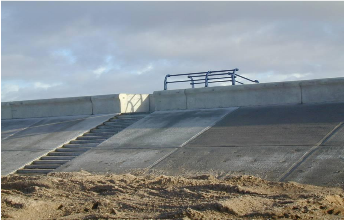
Figure 1.5 : Sloping concrete revetment in front of the sea wall at Southport
