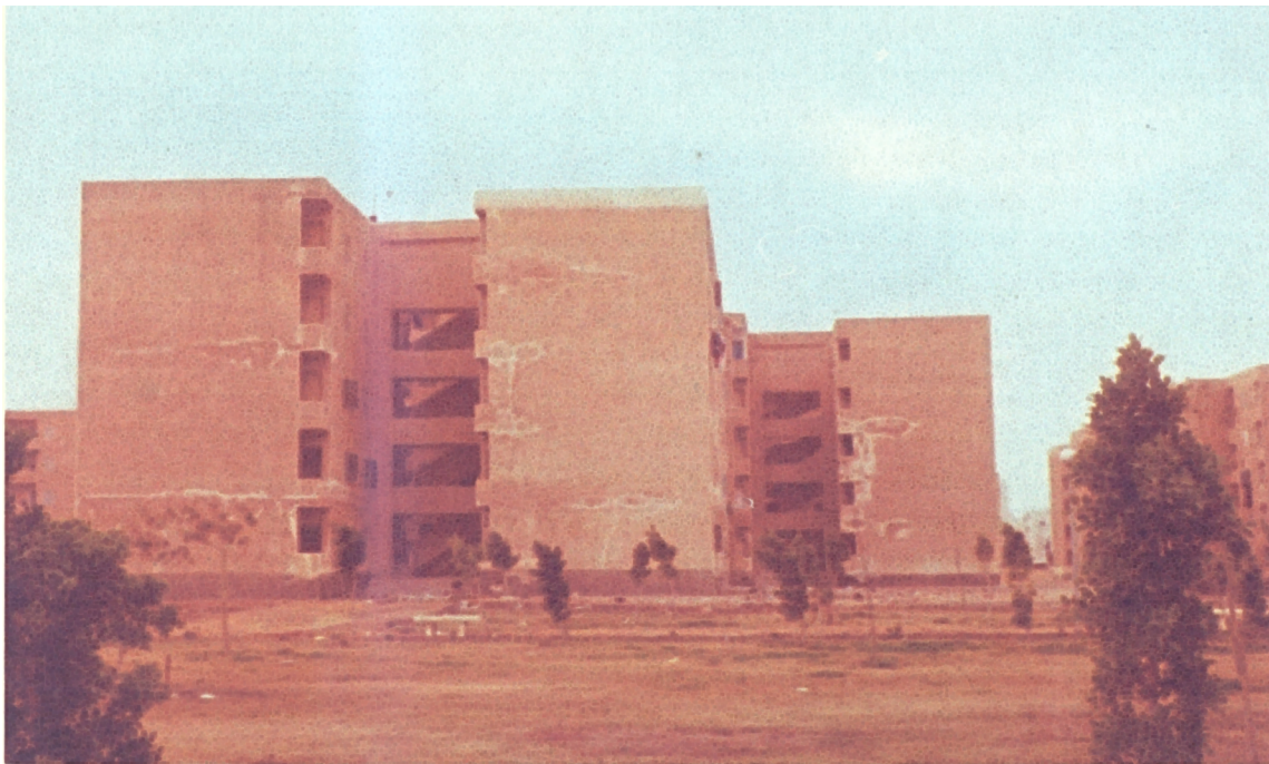
Figure 8.7: Water Leakage on External Walls of Dwelling Buildings in Badr Town. Source: Research Visit to Town, 2002.
