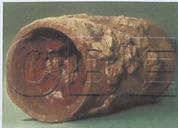
Figure 5.2 Badly corroded pipe from a water distribution system, Courtesy, C. Abernathy, A. Camper
