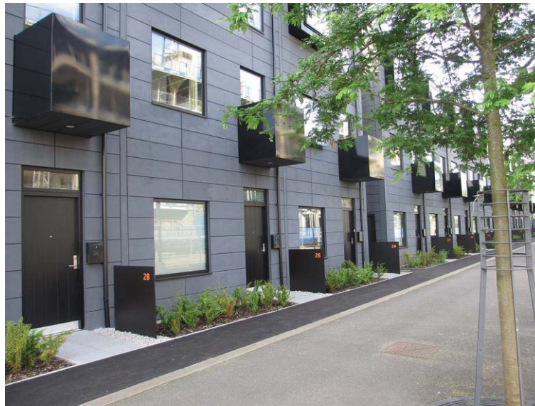
Figure 4. Setting the terrace back from the public realm, and the inclusion of planting, screens and projecting balconies over the entrance, reinforces the sense of threshold for ShedKM's hoUSes.
