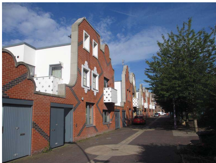
Figure 2. Islington Square, Manchester. External front yards are hidden from view by timber screens, lending the terrace a mews-like quality.
