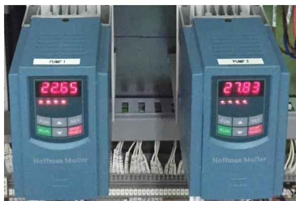
Figure 3.14: Hoffman Muller inverter used to control both pumps' speed.
