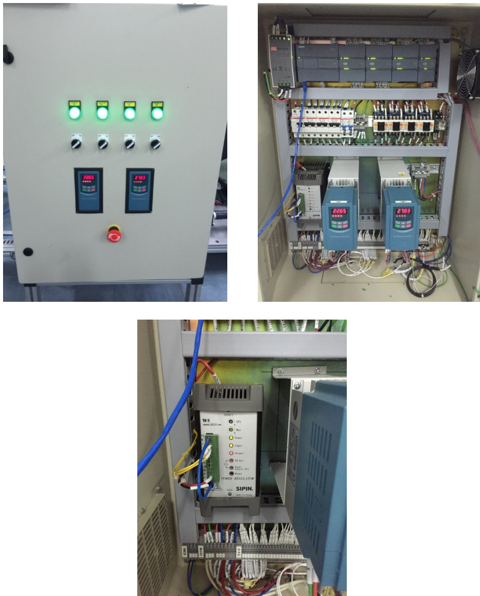
Figure 3.23: Photograph of the PLC system attached with the scada system.
