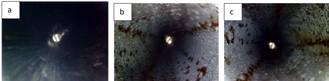
Figure 7.28: Deposition on test section surface under effect of air velocity input [(a) clean pipe surface, (b) 0.0 m/s air velocity & (c) 0.3 m/s air velocity], at constant \Delta T = 15^\circ\text{C} , 0.2 m/s water flow and 500 mg/l concentration .
