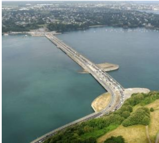
Figure 3-6: La Rance tidal barrage in Brittany France (EDF, 2019)
