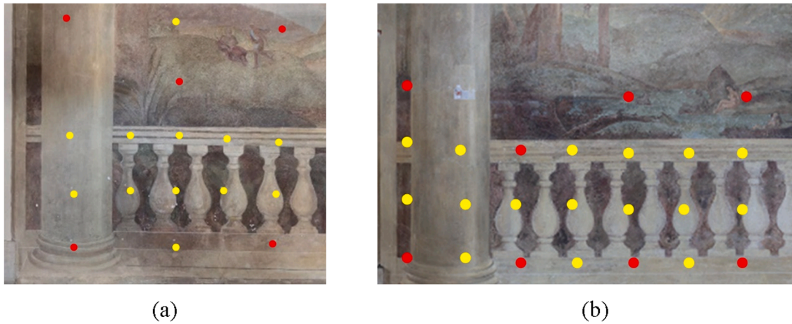
Fig. 7. The sketch of reference point distribution used for image orientation with natural points measured by Total Station (control points – red, check points – yellow) for (a) Test Site I and (b) Test Site II.
