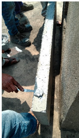
Figure 14. Application of grouting material.
