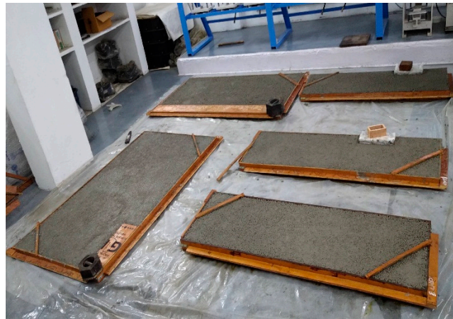
Figure 12. Casting of prefabricated panels.
