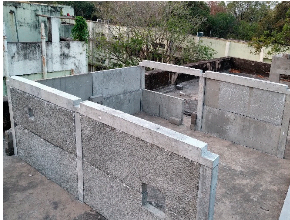
Figure 13. Erection of prefabricated elements.
