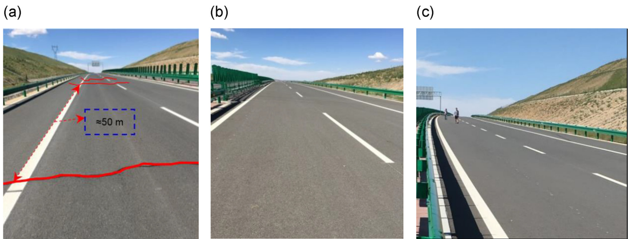
Fig. 5. Appearance of test roads (Li et al., 2018a). (a) SBS MA compared road. (b) LDHs MA test road. (c) SS-LDHs MA test road.
