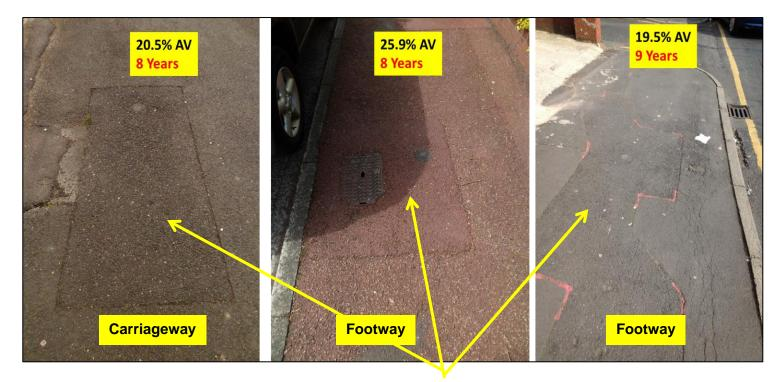
Figure 9: Visual in-situ performance of different reinstatement containing non-compliant AV
