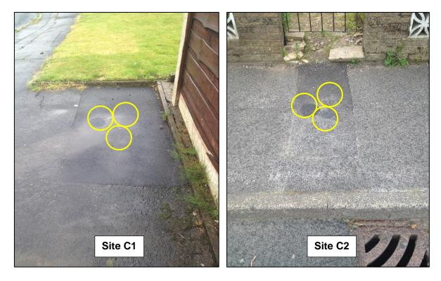
Figure 1: Location of three cores taken by Lab A, Lab B and Lab C from site C1 and C2
