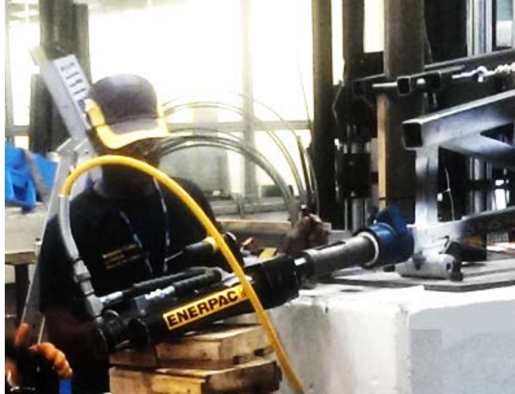
Fig. 6: Prestressing of cable
