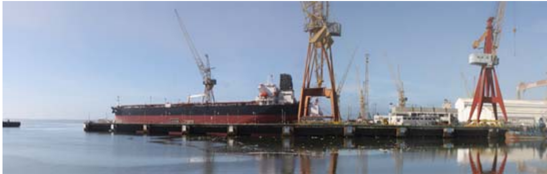
Figure 1 - View of the Quay 3.
