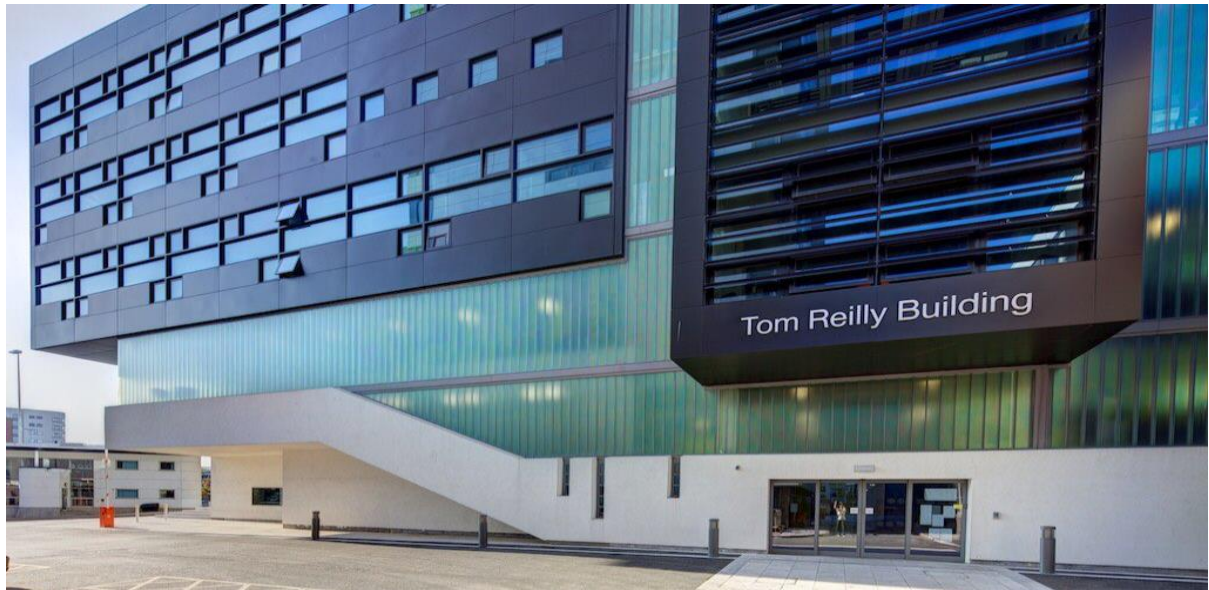
Figure 4. The Tom Reilly Building (TRB), Liverpool John Moores University. Facilities within the TRB were used for data collection of Chapters 4 and 6.
