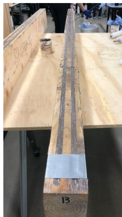
c) Installed NSM FRP bar (Step 4)
