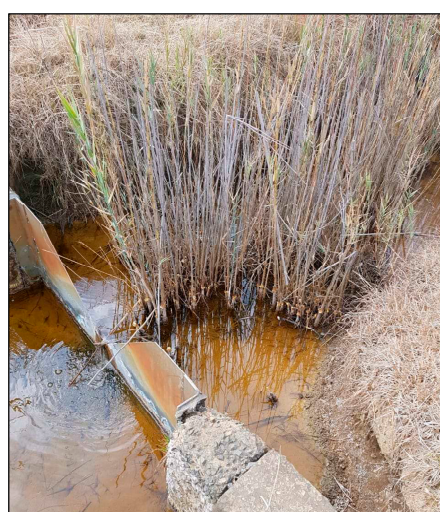
Figure 1. Overflow weir—AMD collection point.
