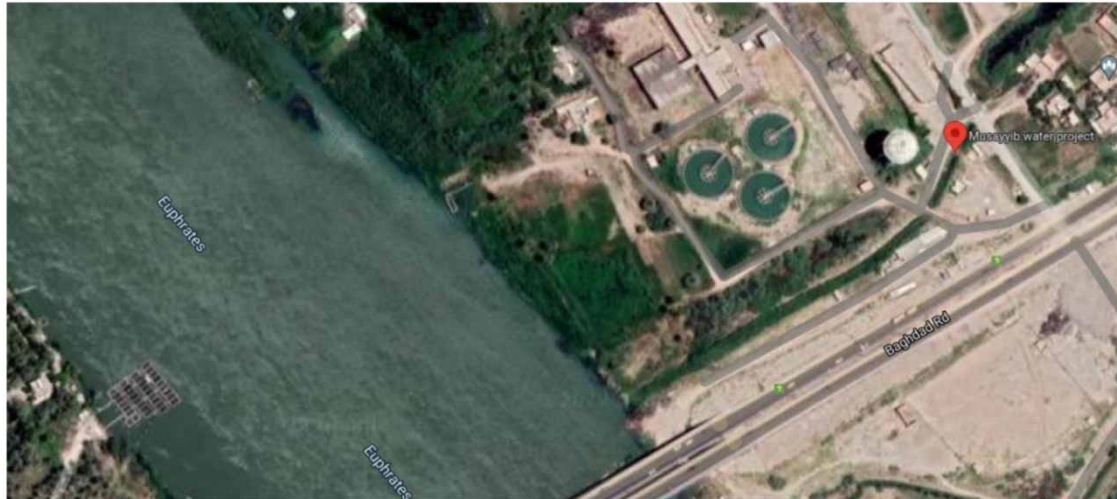
Figure 1 | Al-Mussaib water treatment plant.
