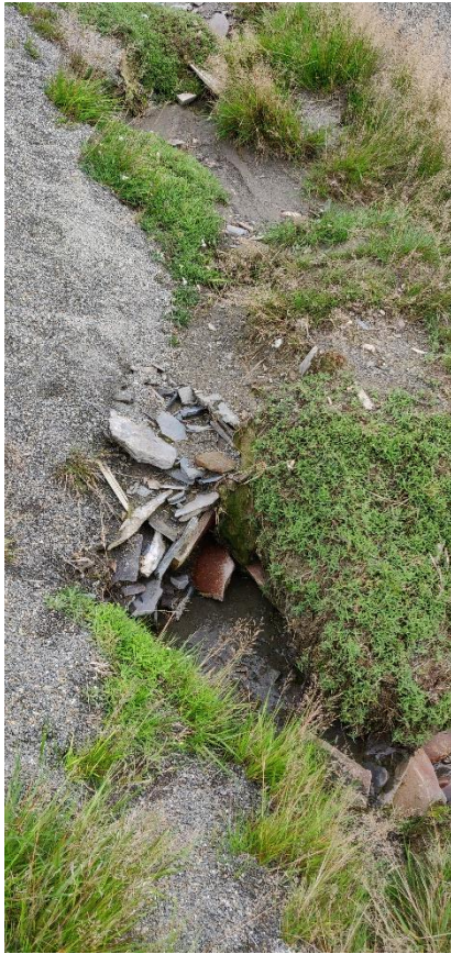
Figure A2. Dry channel at Mill Race Stream with evidence of an output from subsurface flow in the lower area.
