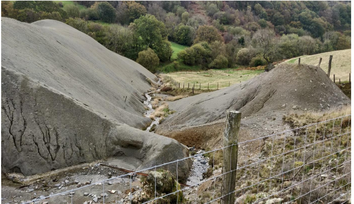
Figure 3. Main spoil heap at Wemyss mine. High sided spoil slopes down towards Mill Race Stream, flowing through the centre.
