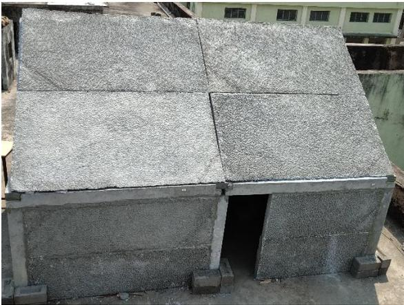
**Figure 26.** Erection of slab panels
