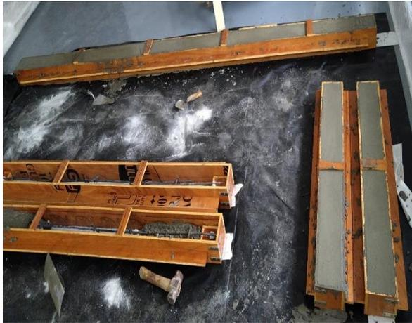
**Figure 17.** Casting of structural elements
