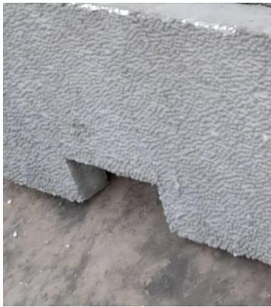
**Figure 19.** Provision for window opening
