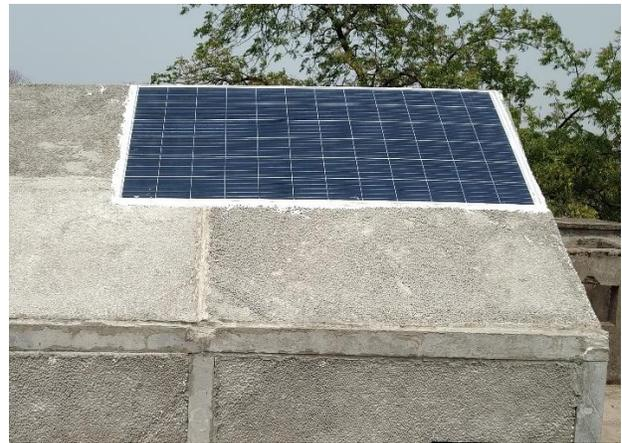
**Figure 27.** PV panel embedded into roof
