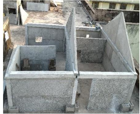
**Figure 25.** Erection of roof supporting elements
