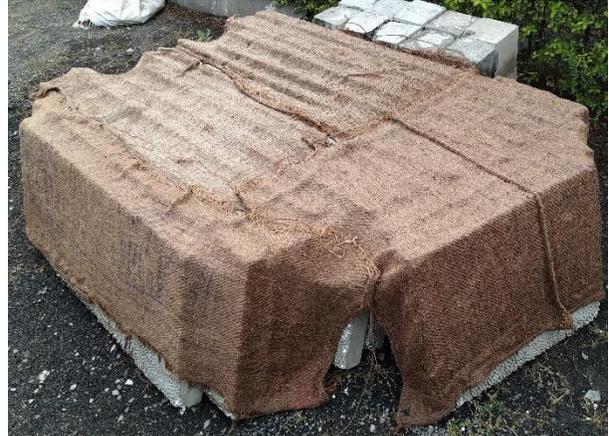
**Figure 22.** Curing and stacking of prefab panels
