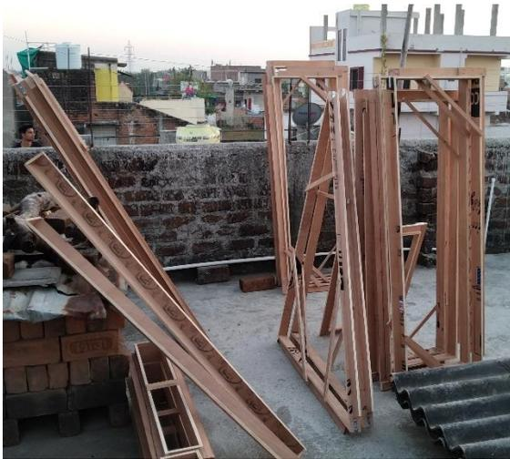
**Figure 15.** Wooden moulds
