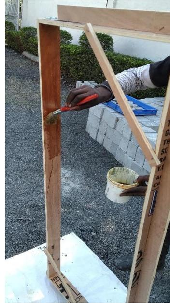
**Figure 16.** Oiling of moulds
