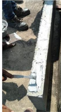
**Figure 24.** Application of Epoxy grout
