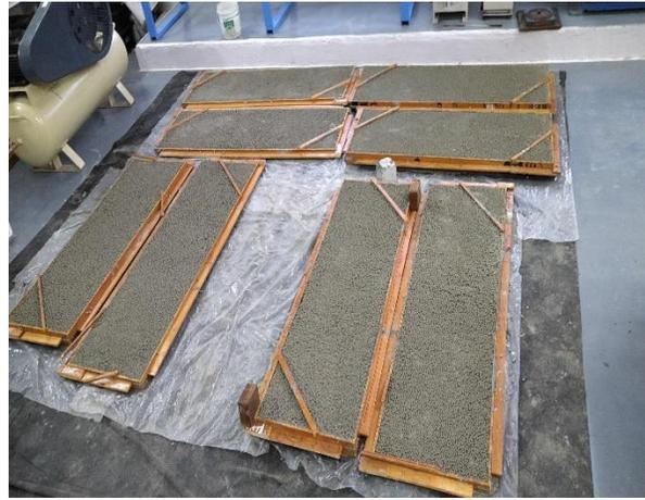
**Figure 18.** Casting of prefab panels
