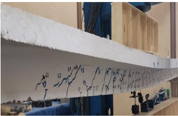
Fig. 15. Crack pattern of OWRS5
