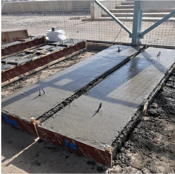
Fig. 5. Concrete casting of the specimens.
