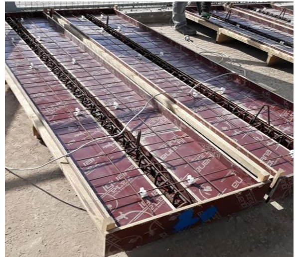
Fig. 4. Wood formwork and reinforcement of the specimens
