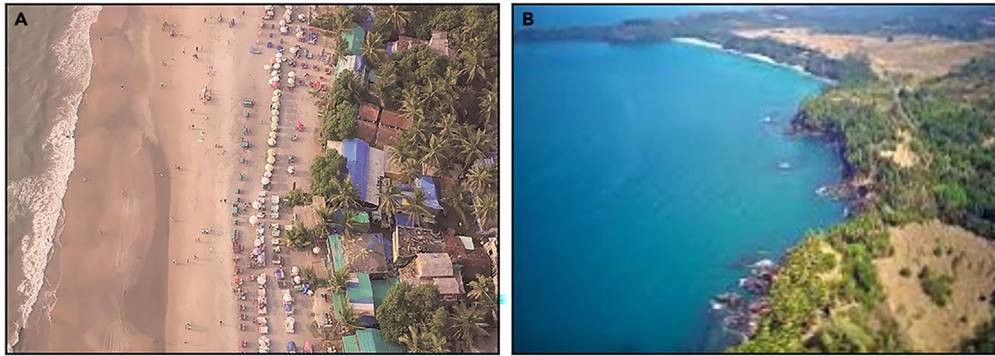
Figure 8. Drone images of coastal stretches of the study area (A) Sandy coast and (B) cliffed coast.
