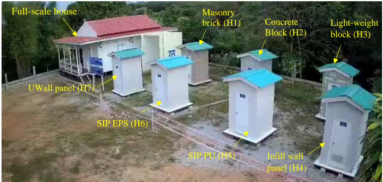
Fig 7. Full-scale house by Hybrid wall panel and Scaled-down house units built with: (a) Mon blocks (H1), (b) brick blocks (H2), (c) LW blocks (H3), (d) composite infill wall panel (H4), (e) SIP PU (H5), (f) SIP EPS (H6), and (g) UWall panel (H7).
