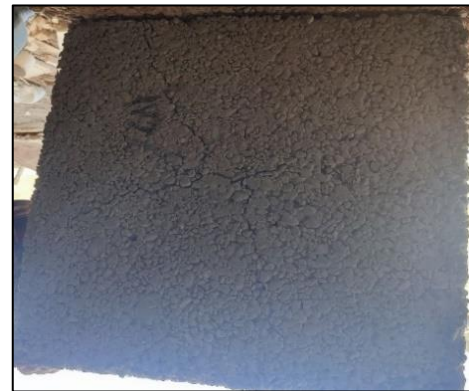
Figure 15. Crack pattern at failure of 0.75 % PP specimen
