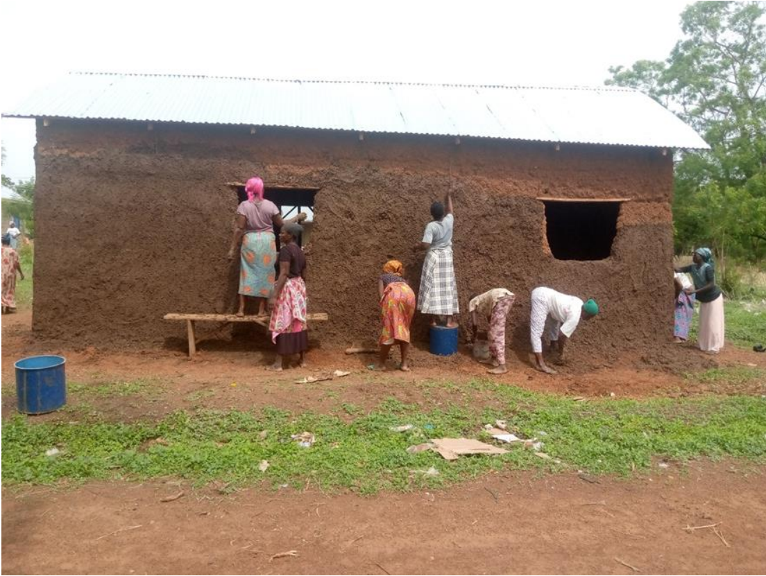
Figure 2: Women plastering a newly constructed earth house in Tamale.
