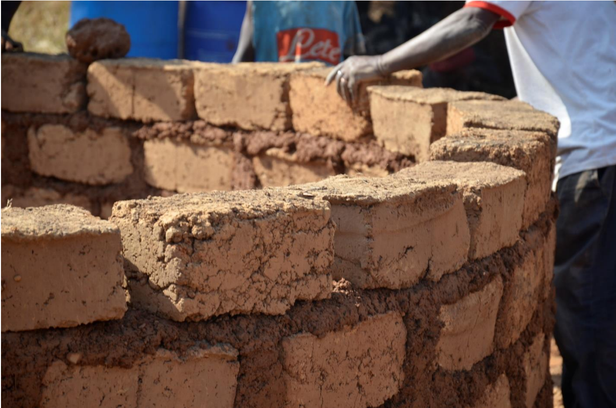
Figure 3: A man demonstrating the construction of a building using sundried earth bricks and earth mortar joints in Wa
