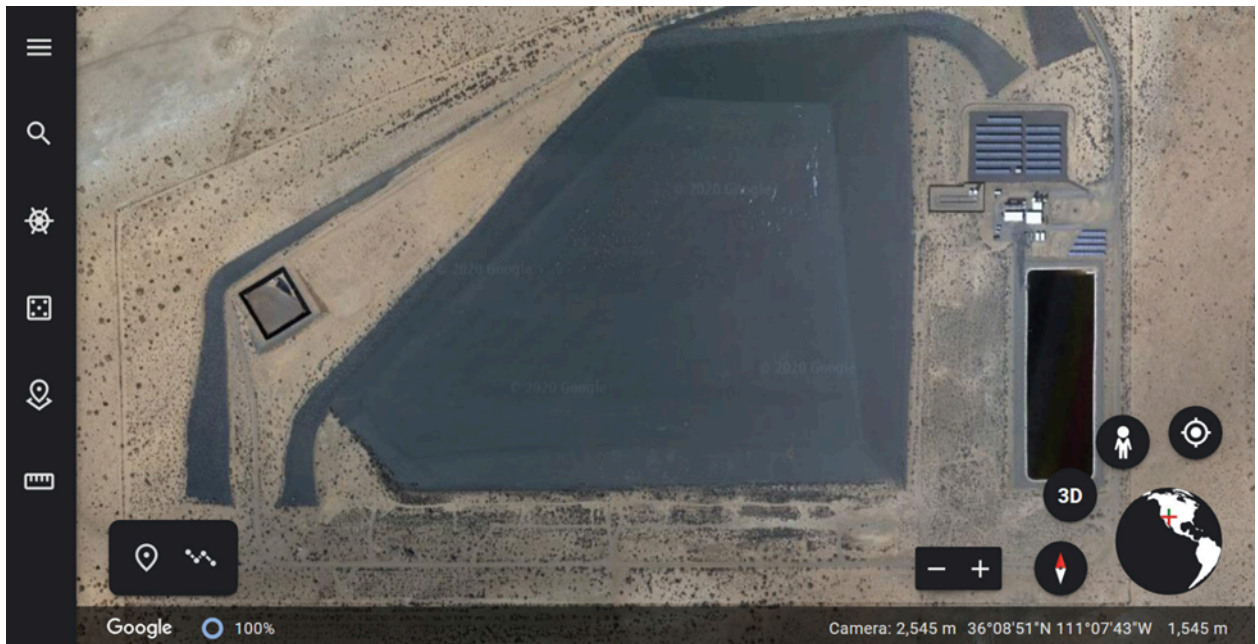
[Tuba City, Arizona, Uranium Disposal Cell - contaminated materials capped in concrete on Navajo land - Source: Google Earth. Included via Google Earth attribution guidelines]
