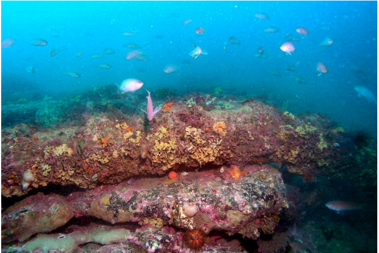
Figure 12. The BassLink cable (Tasmania, Australia), protected by a cast-iron half-shell, showing a heavy encrustation of algal and invertebrate species on the underlying basalt reef.
