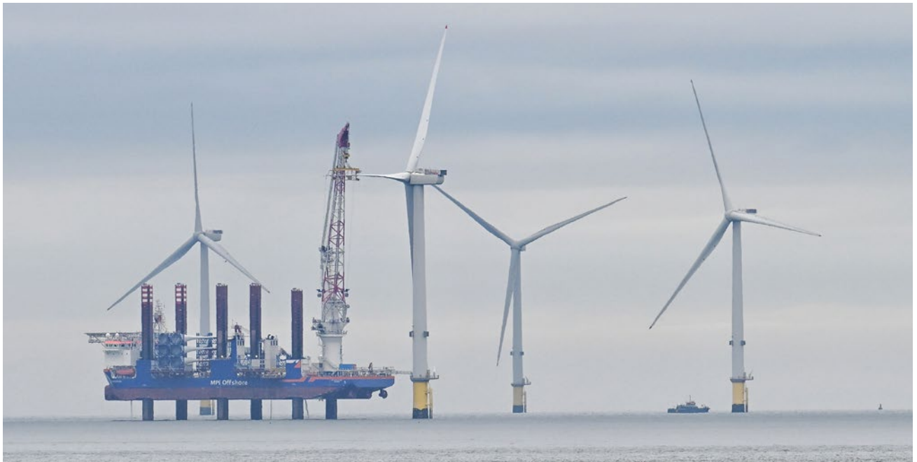
Figure 6. Windfarm near Hilbre Island, United Kingdom.
