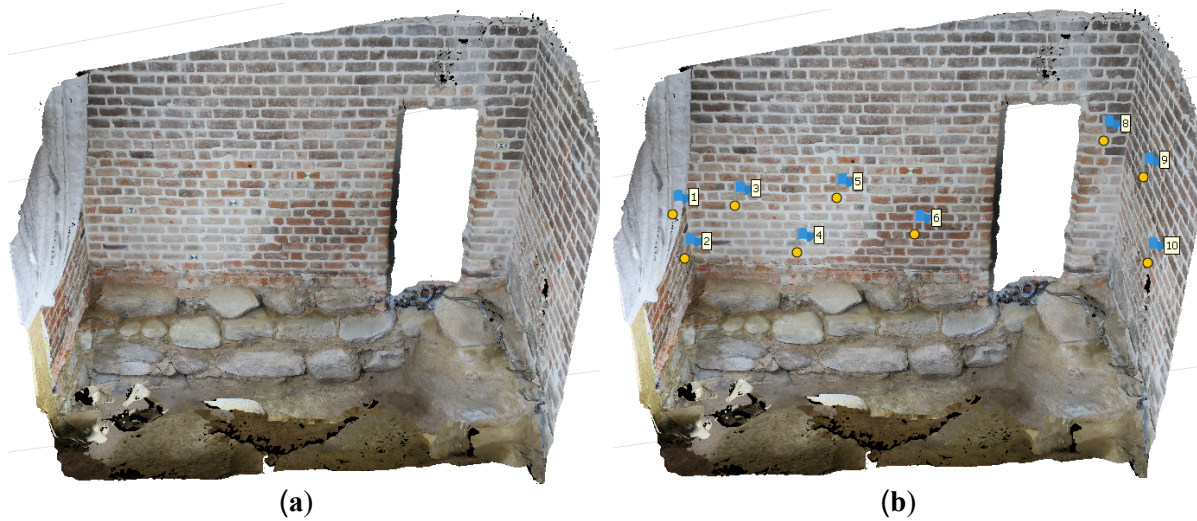
Figure 3. The textured model of the basement during the first excavation stage: (a) the resulting model, (b) with marked reference points. - Epoch 1.
