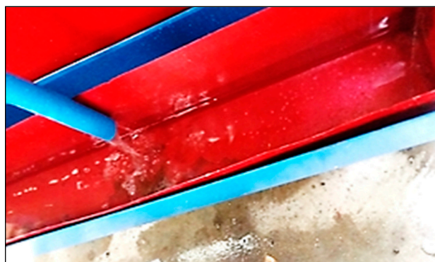
Figure 11. Steel container to collect runoff [15].
