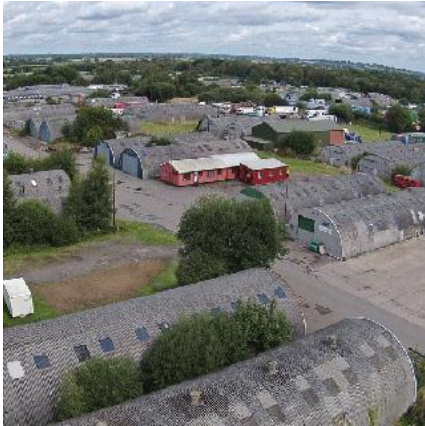
Fig 4.1d: Wem Industrial Estate (Bulleys Bradbury, 2019)
