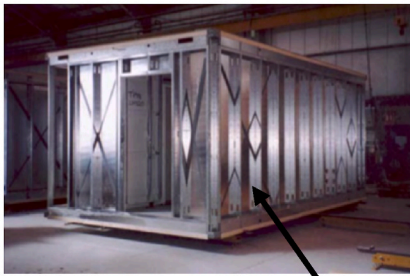
Side walls constructed from C-section posts
