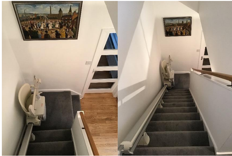
Figure 3.2. Photograph of the location where the stair fall occurred (Faller-Female2, aged 70-79). The image highlights the absence of a continuous handrail and the restricted corner space created by the stair lift installation, both of which may have contributed to the fall.
