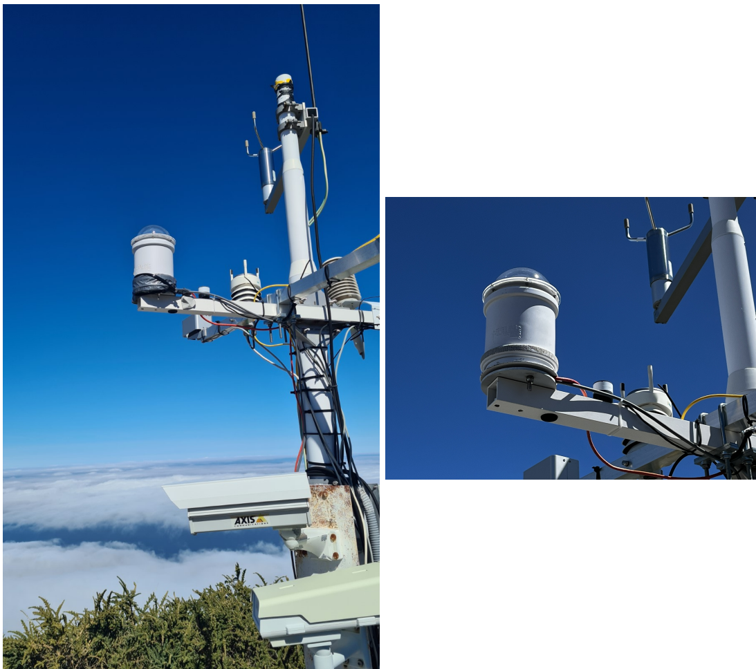
FIGURE 3.13: Skycam O installed on the weather mast at the Liverpool Telescope. The camera is housed in a weatherproof enclosure and connected to the observatory network for real-time data transmission.
