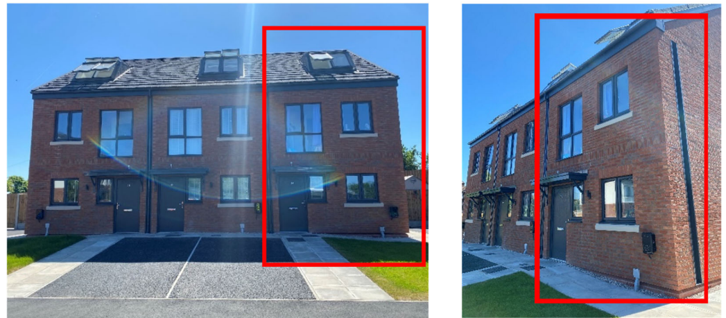
Figure 3. Brooklands Building, Wirral Waters, UK. The red boxes highlight the selected dwelling analysed in this study. Photo: Deelaram Nangir.
