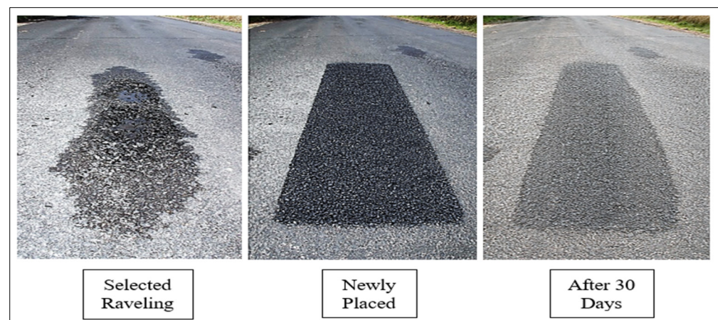
Figure 17. Field Repair of Pavement Raveling using the Developed Most Suitable SC-WMA.
