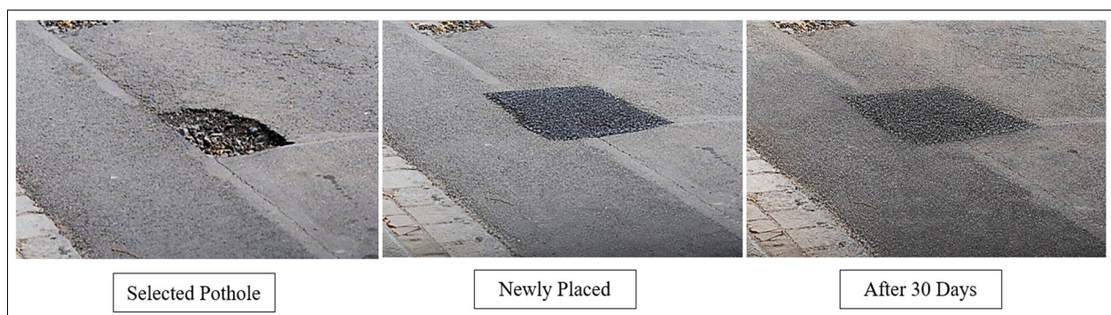
Figure 15. Field Repair of a Pothole using the Developed Most Suitable SC-WMA.
