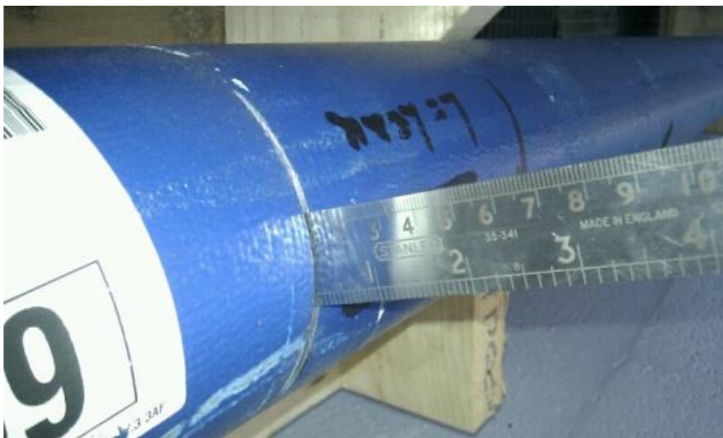
Figure 64: Leakage from the Ø118mm pipe
