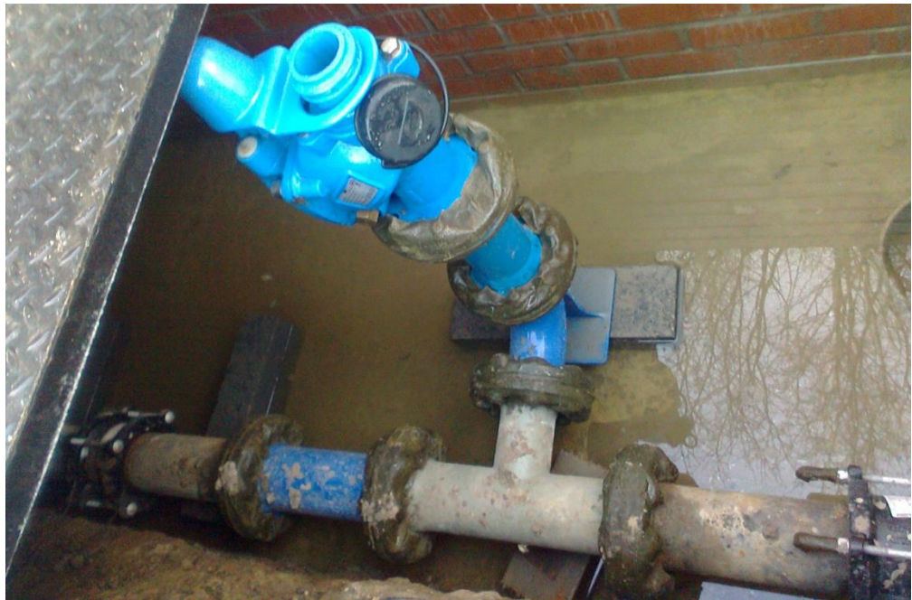
Figure 45: Access valve in the Worthington UU test site
