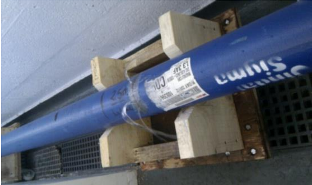
Figure 63: Crack to simulate leak
