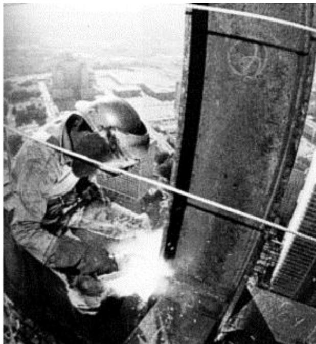
Figure 3: Representation of Arc welding
